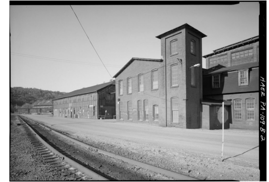
Cambria Iron Company, Pattern Shop, ~1968-69
